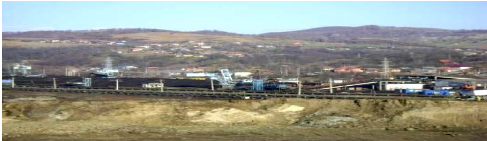
Fig. 6. The belt conveyance, coal handling has an impact on the air through particulate emissions in suspension
