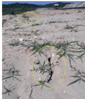
Fig. 3. Cracks on the berm of second step of the inner dump
