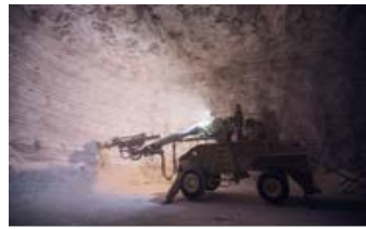
Fig. 6. SECOMA perforation installation
