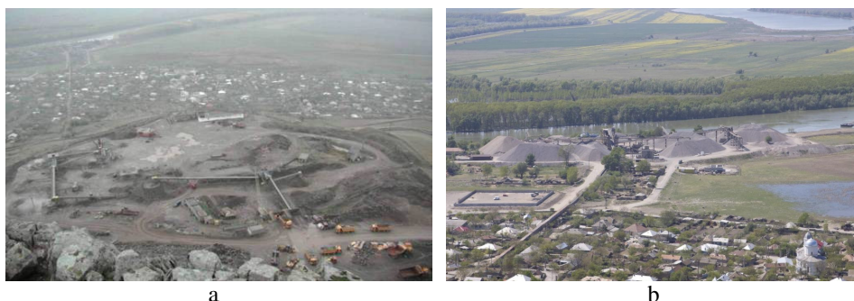
Fig. 2. Crushing plant and loading dock
